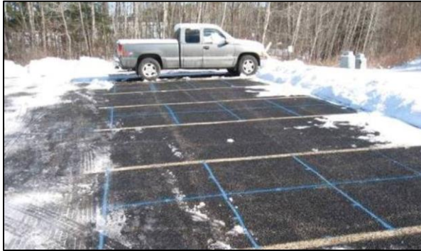
Figure 5 - Porous asphalt (left) and dense mixed asphalt (right) parking lots shown one hour after plowing on a 25° F day in February, 2007. Source: University of New Hampshire Stormwater Center
