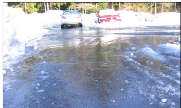
Figure 6 - Porous asphalt (left) and dense mixed asphalt (right) parking lots shown after a spring rain on snow event Source: University of New Hampshire Stormwater Center
